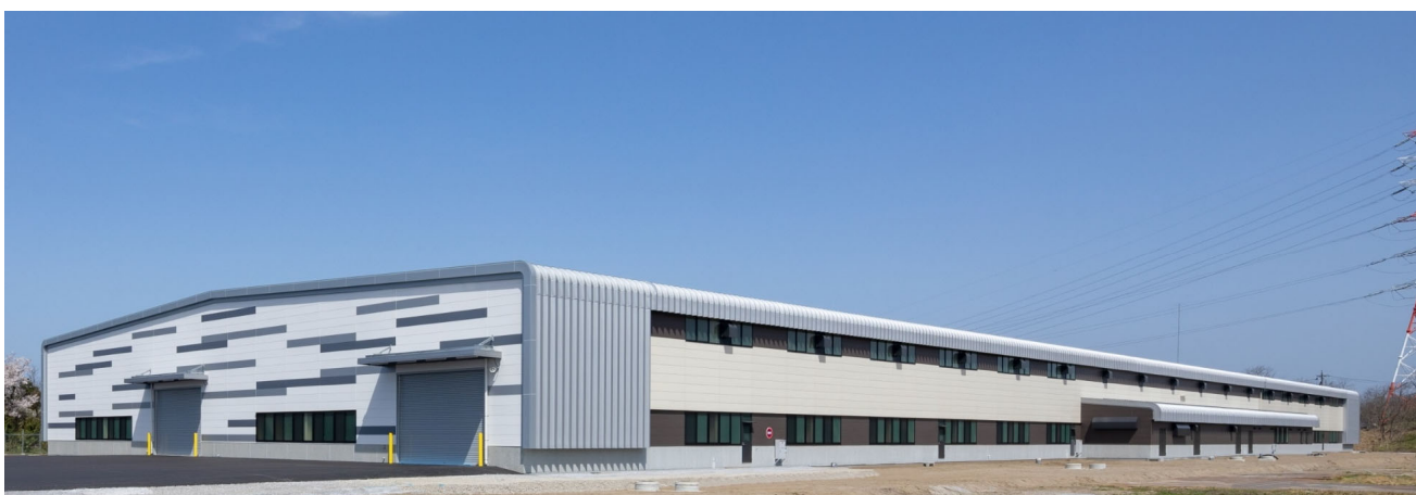
Fukui Yodoko No.2 Plant (No.1 Building)
