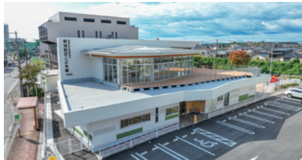
A building with the YODO fire-proof panel Barrier Lock Hyper (Chromate-free specification)
