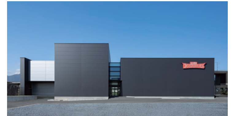
The YODO fire-proof panel Grand Wall is used at the Kobelco Kobesteelers Nadahama Clubhouse
