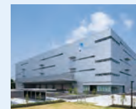
YODO fire-proof panel Grand Wall installation example
