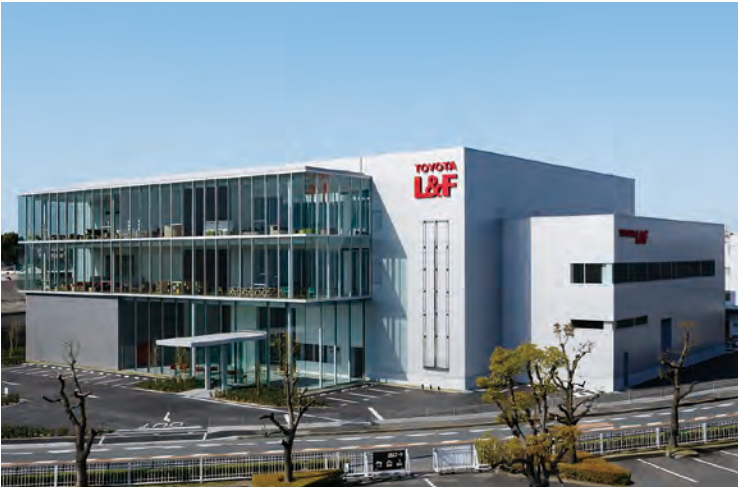
YODO fire-proof panel Grand Wall installation example
