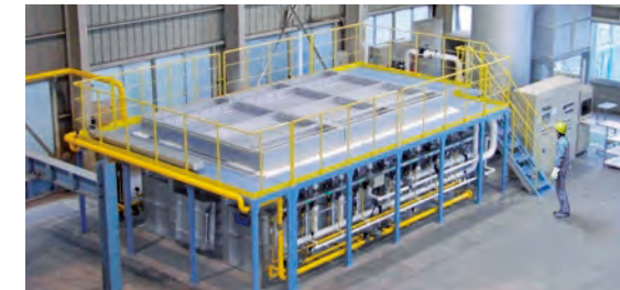
Fire-proof and Fire-resistance Test Equipment (Osaka Plant)
