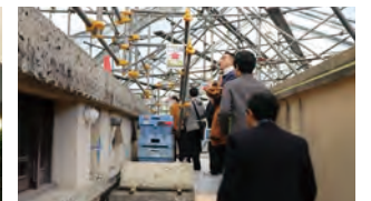
A tour during construction
