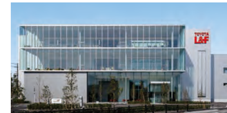
YODO fire-proof panel Grand Wall installation example
