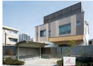
Renovating former sites for employee housing and repurposing them as daycare centers
