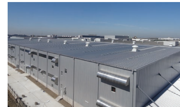
Installation example at Yodoko Building Materials (Hangzhou), China 66H roofing and 806 siding Building name: Hitachi Transport System (Tianjin) New No. 2 Warehouse
