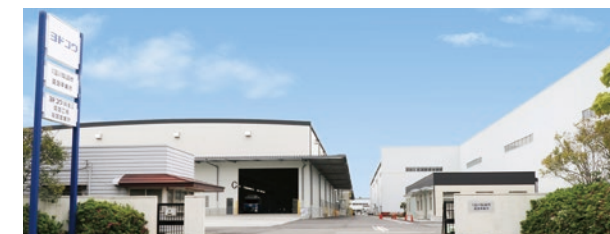
Himeji Plant production site for YODO fire-proof panel Grand Wall
