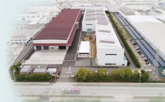
Full view of the Himeji Plant
